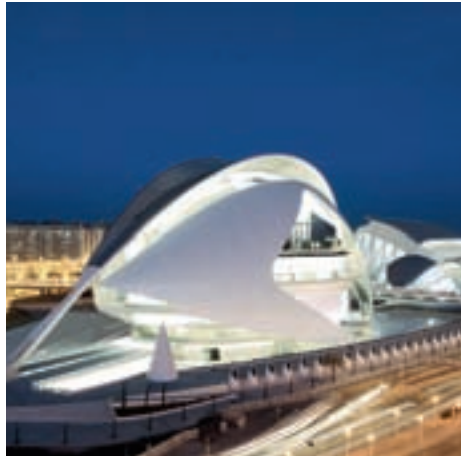
The Palau de Les Arts in Valencia – one of the largest opera houses in the world. The lighting director opted for OSRAM QTl DALI control gear for its outstanding performance.
